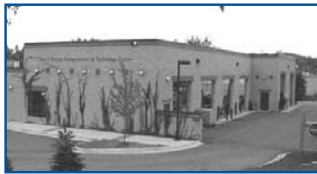
Transportation center and garage
