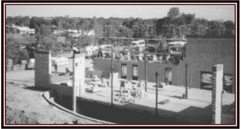
New Transportation Center takes shape
